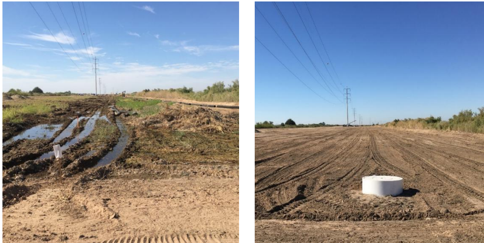
Seepage Recovery Project, Before and After
