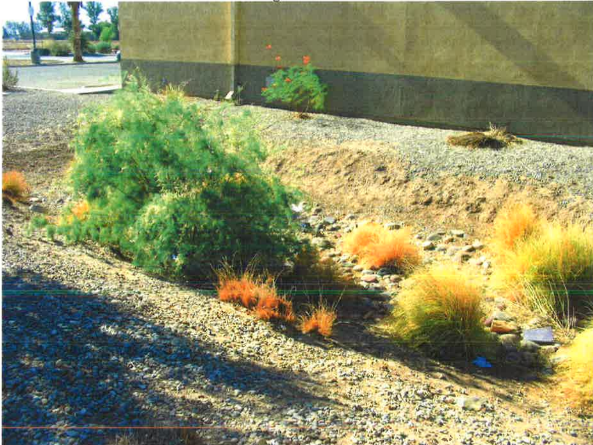
Landscaped drainage facility/detention basin, immediately north of the UETA Duty Free store, facing southeast
