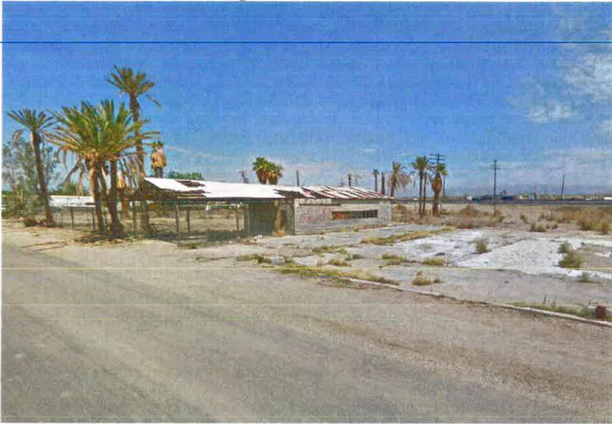
Abandoned structure and vacant lots on E 1 st Street, facing north west.
