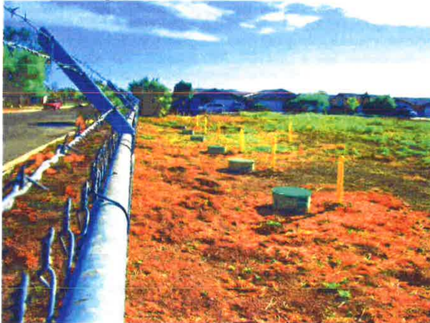
Existing wastewater facility with leach field, looking south on Poe Colonia Road
