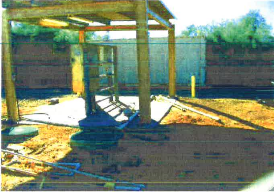
Existing wastewater facilities located along Poe Colonia Road
