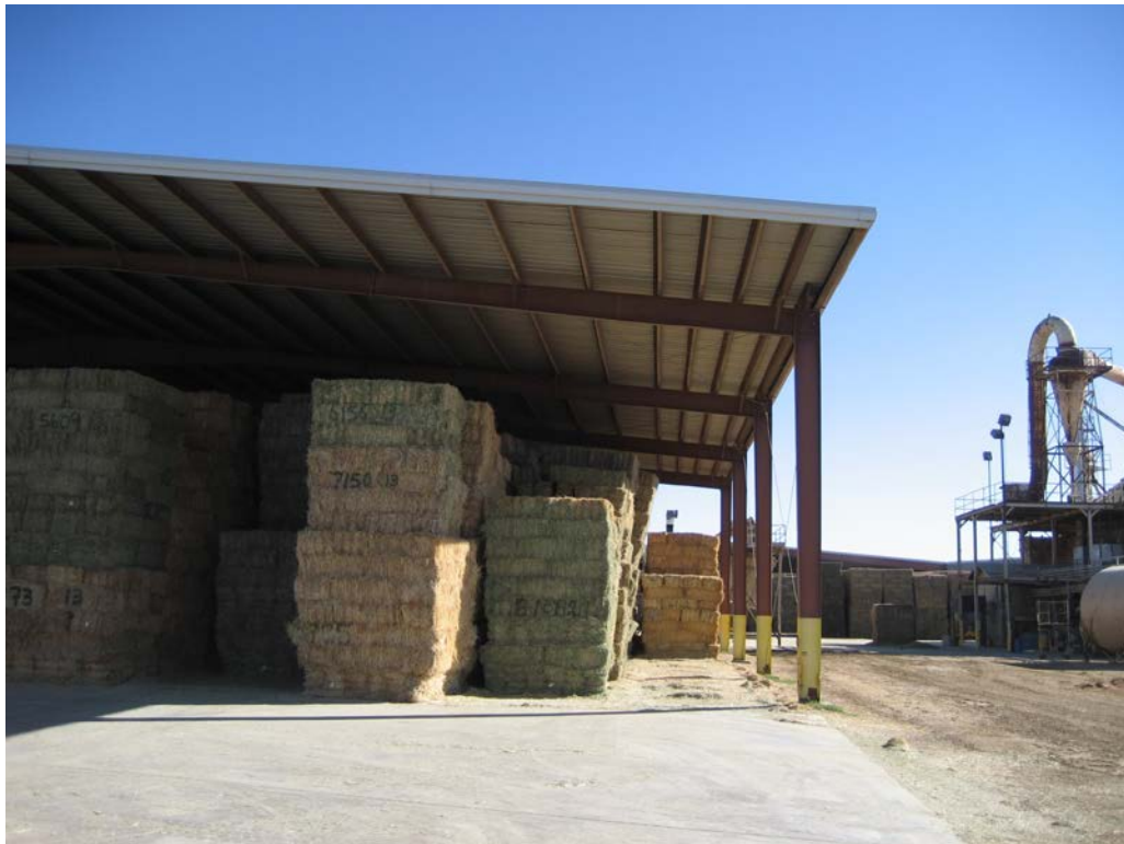
View of typical hay barn [seven (7) onsite] 100- feet of separation between hay barns
